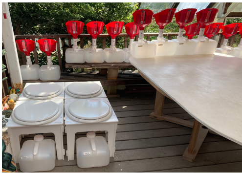
Waterless unisex “Cubie” Urinals and “Pee-Toilets”
