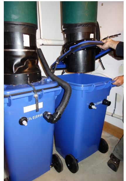
Fig. 2. Installation of new empty bin to chute
