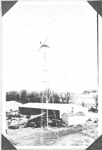
PHOTO 14. Air Electric 2000 Watt - 32 Volt - On Tower
